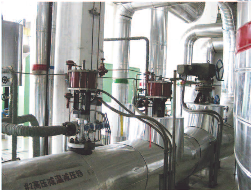
CIRCOR lancer desuperheater installed at power plant
